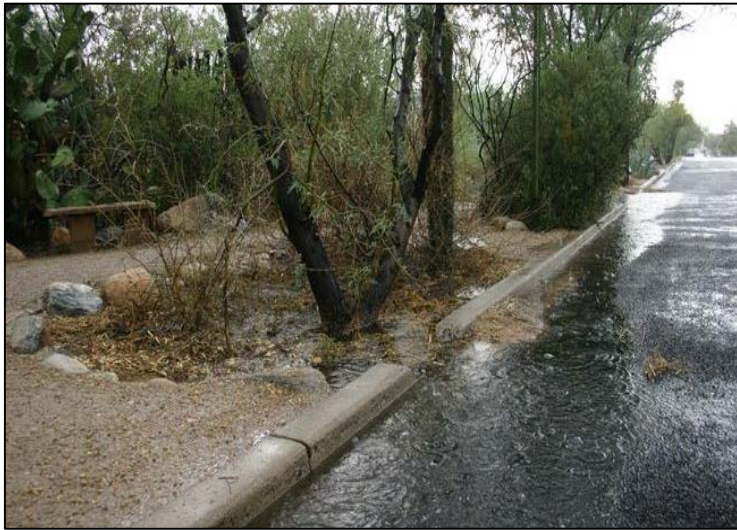
Green infrastructure with curb cut (Lancaster, 2015)
