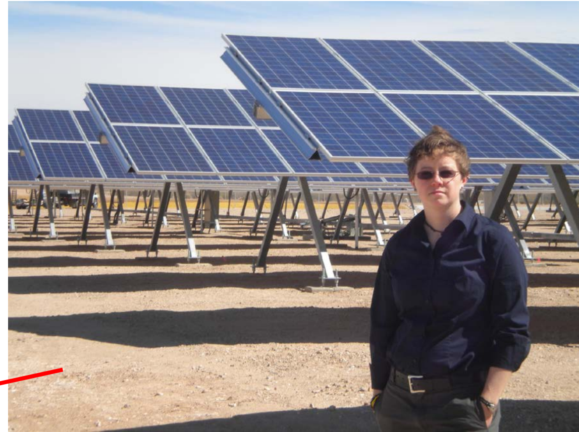
1.2 MW (utility-scale) PV power plant “Solon 1” at UA Science and Tech Park
